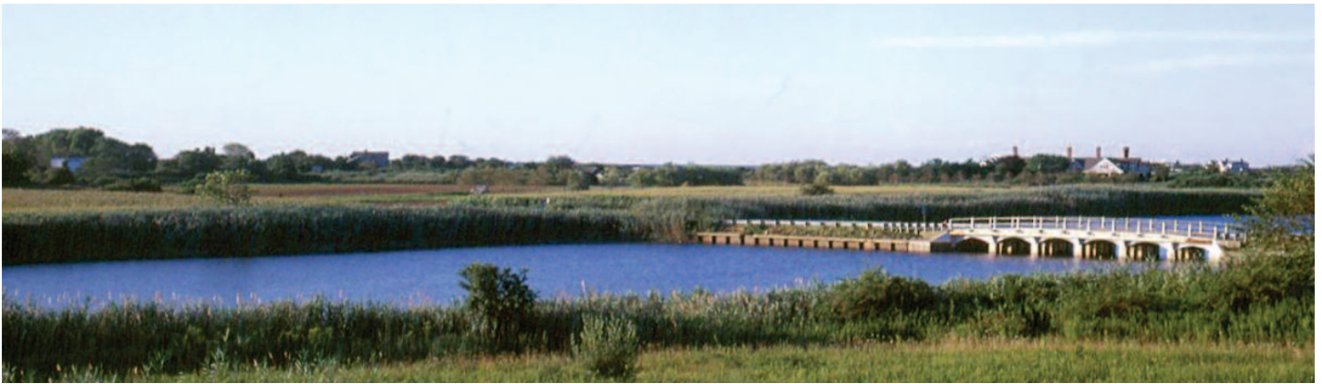
The White's Golf Lot property is located to the left of Sagg Bridge.
